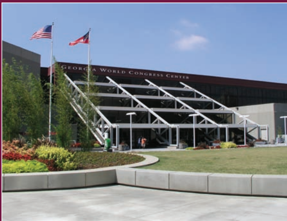
Exterior view of the Georgia World Congress Center, the premier convention and conference center in the Southeastern U.S.
